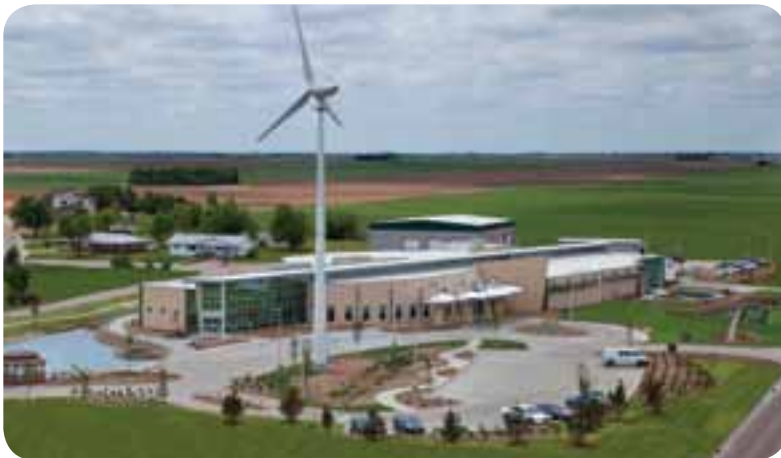
Construction of the new Kiowa County Memorial Hospital was completed in March. Featuring a wind turbine, it is 32 percent more energy efficient than the old facility. photo by Steve Rasmussen
