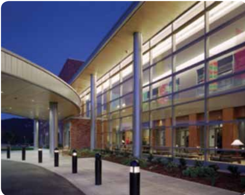
When Providence Newberg Medical Center in Newberg, Ore., was rebuilt in 2006, it became the first LEED gold certified hospital in the country.
