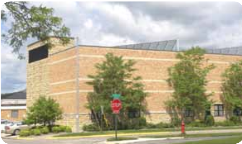
Prairie du Chien Memorial Hospital in Prairie du Chien, Wis., has undergone several green renovations since 2008, including the installation of solar panels on the roof of the 53-year-old building.
